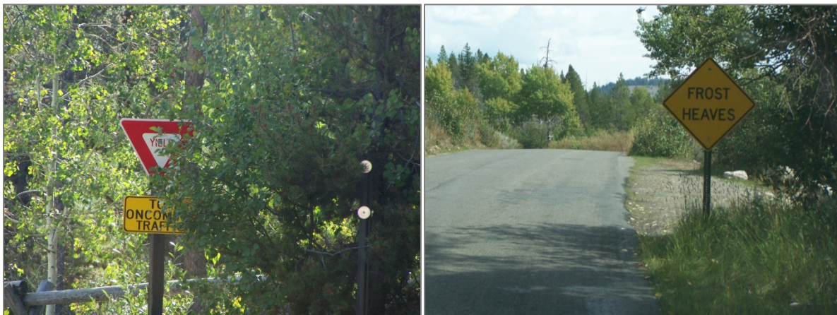
Figure 4. Obscured and Confusing Signs
