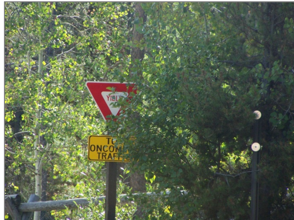
Figure 19. Sign Blocked by Vegetation
